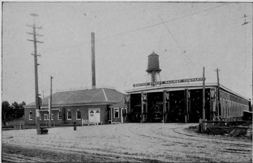
POWER HOUSE AND CAR BARN, HAMPTON, N. H.
