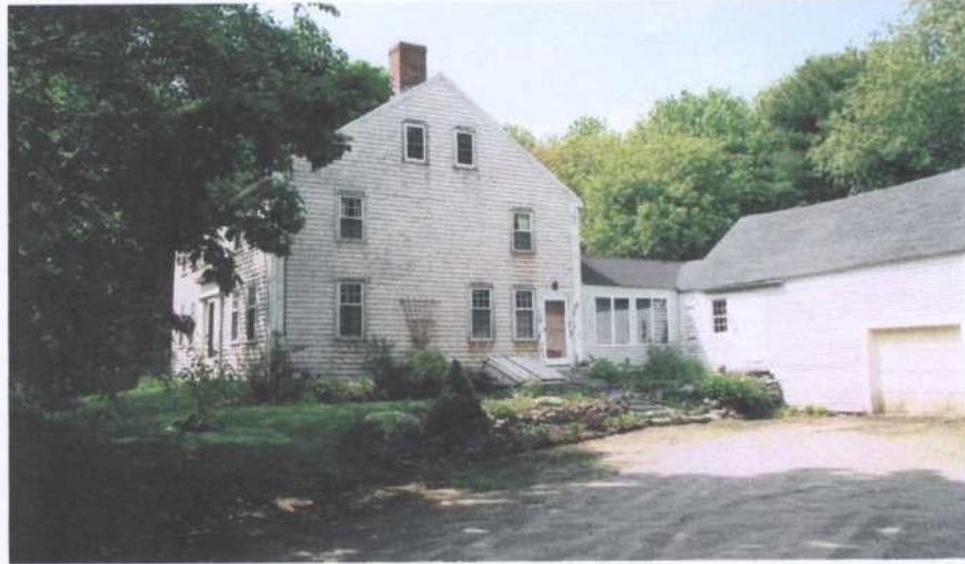
View from right side showing addition to the rear.
